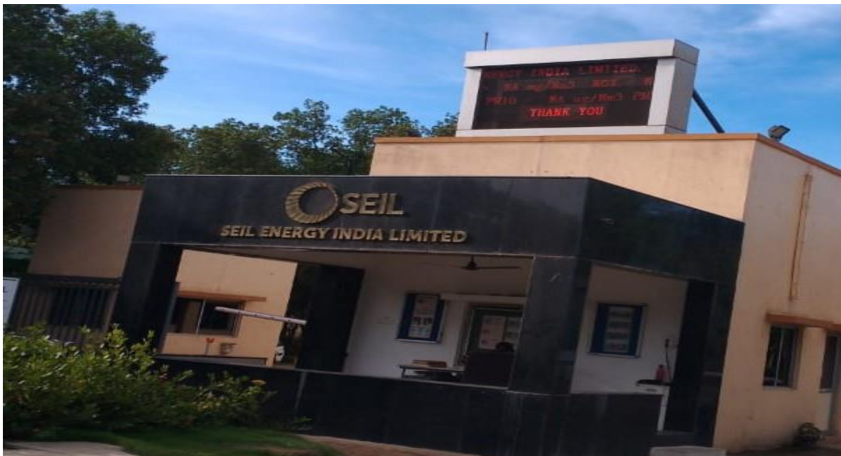
MAIN GATE DISPLAY BOARD - AMBIENT AIR QUALITY, EMISSIONS & HAZ. WASTE DATA DISPLAY
