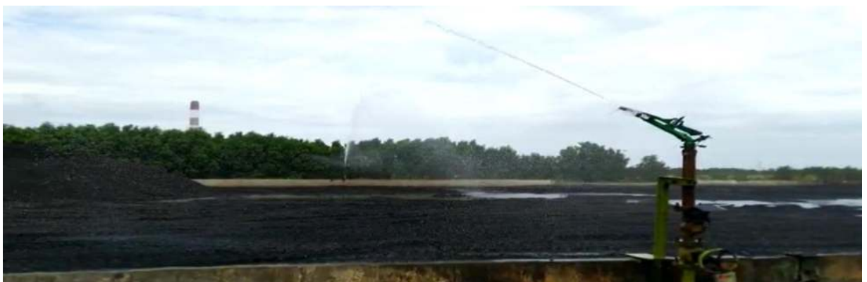
COAL YARD WATER SPRINKLING
